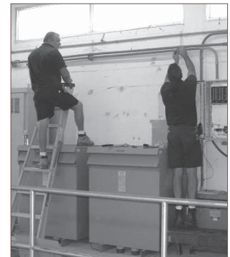
Town public works employees wire a generator.
