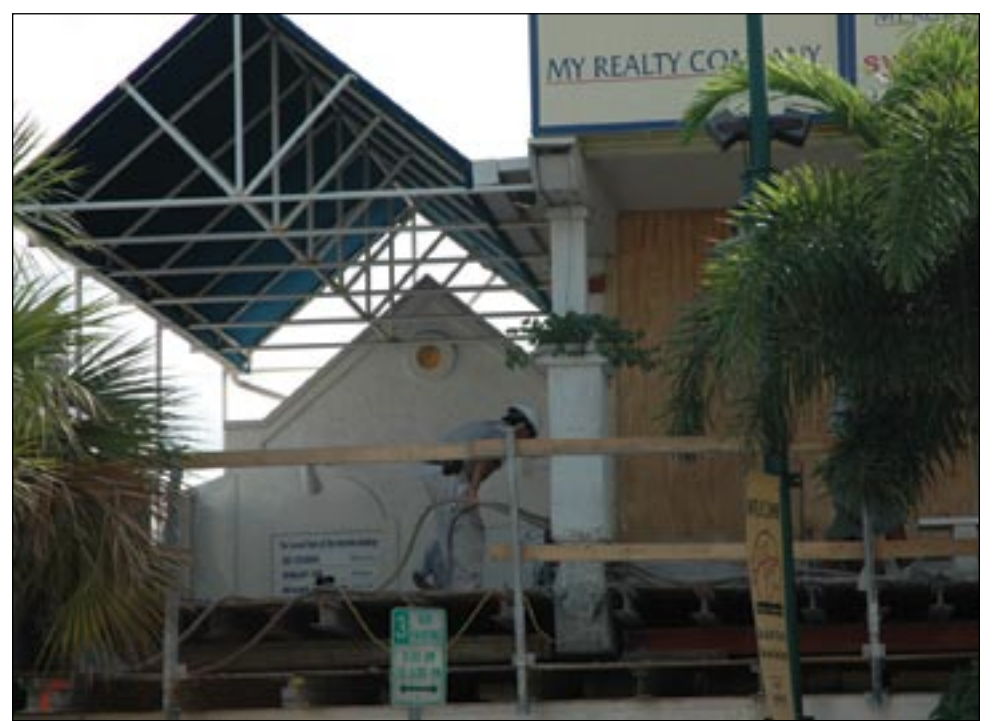
You can see the scaffolding enfolding the front doors and windows.
